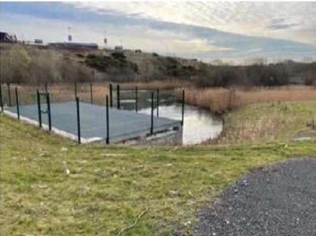
Photo B - Outfall control structure to regulate flows for link road and new development
