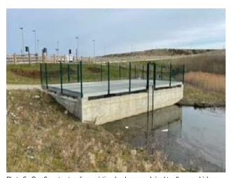
Photo C - Overflow structure from existing developer pond sized to allow new highway flows
