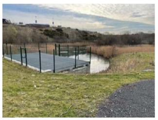
Photo B - Outfall control structure to regulate flows for link road and new development
