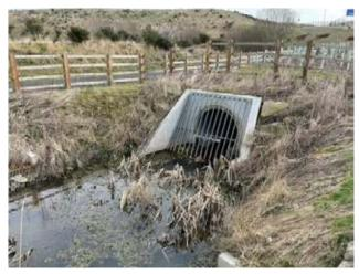
Photo A - Outfall from Culvert under new link road into Carr Beck
