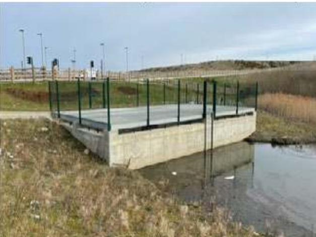
Photo C - Overflow structure from existing developer pond sized to allow new highway flows
