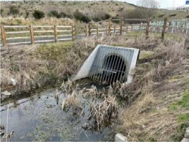
Photo A - Outfall from Culvert under new link road into Carr Beck
